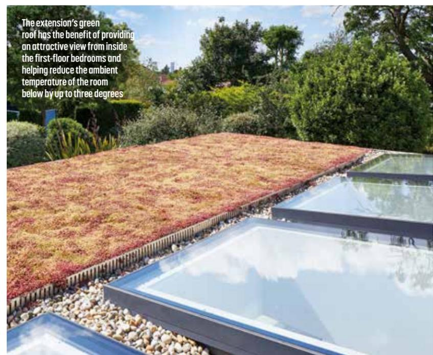
The extension's green roof has the benefit of providing an attractive view from inside the first-floor bedrooms and helping reduce the ambient temperature of the room below by up to three degrees
